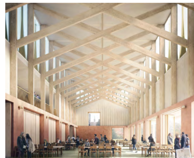
Expressed timber framed construction
