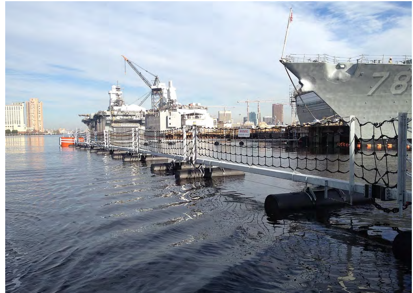
Typical exclusion boom
