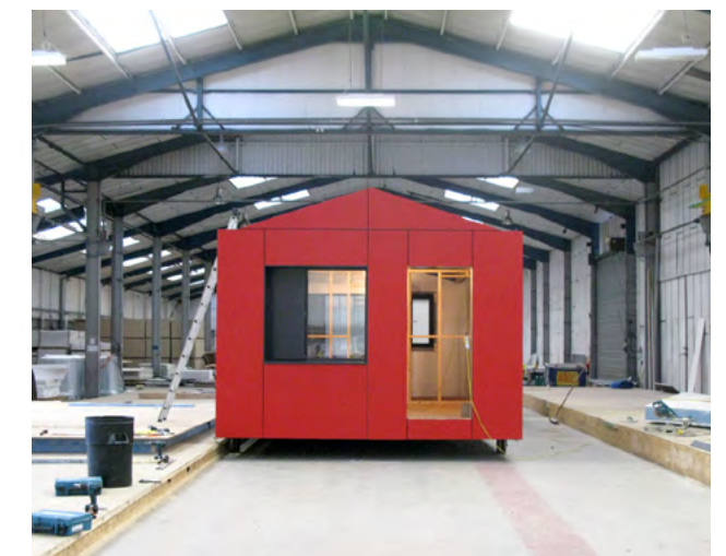
Off-site prefabricated modules
