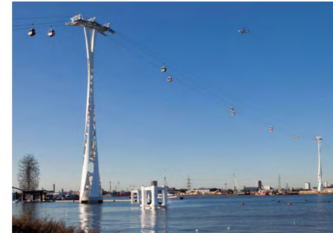
Expedition Engineering Structural Engineers
